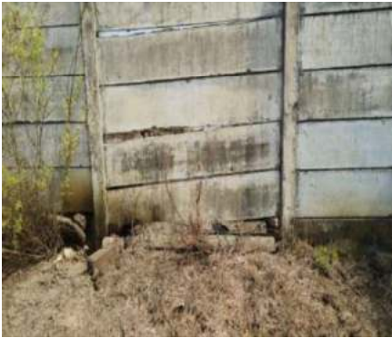
Wet patches of water flow are observed from the unit to agricultural land under cement sheet boundary wall which was observed gone in to nearby agricultural land of other farmer.
